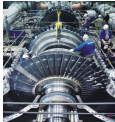
A rotor positioned for final seal clearance check.
