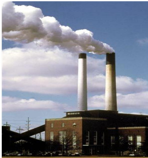
Stateline Power Plant near Hammond, IN
